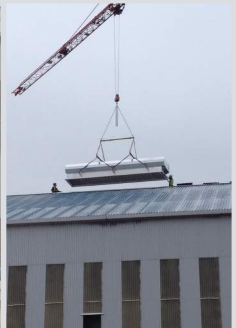
Ventilators being installed on Alcoa's new roof
