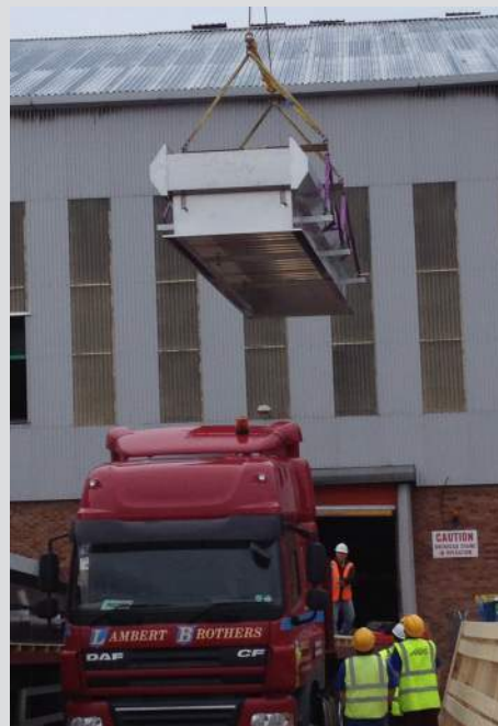
Pre-fabricated Labyrinth natural ventilators
